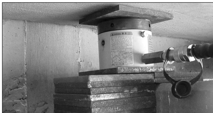
Figure 5, Typical Velocity Fuse Installation
